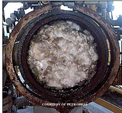
Figure 1 – Hydrate blockage in pipeline
