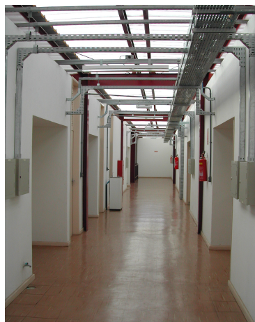
Figure 3 (b). View of the hall
