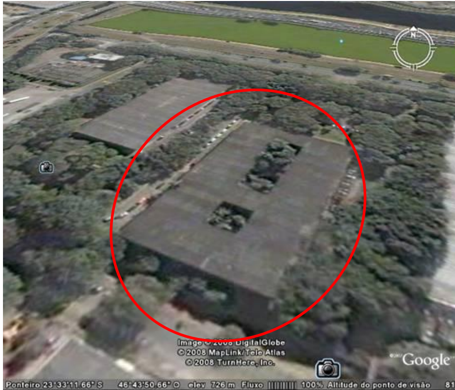
Figure 1. Aerial view of the Mechanical Engineering Building
