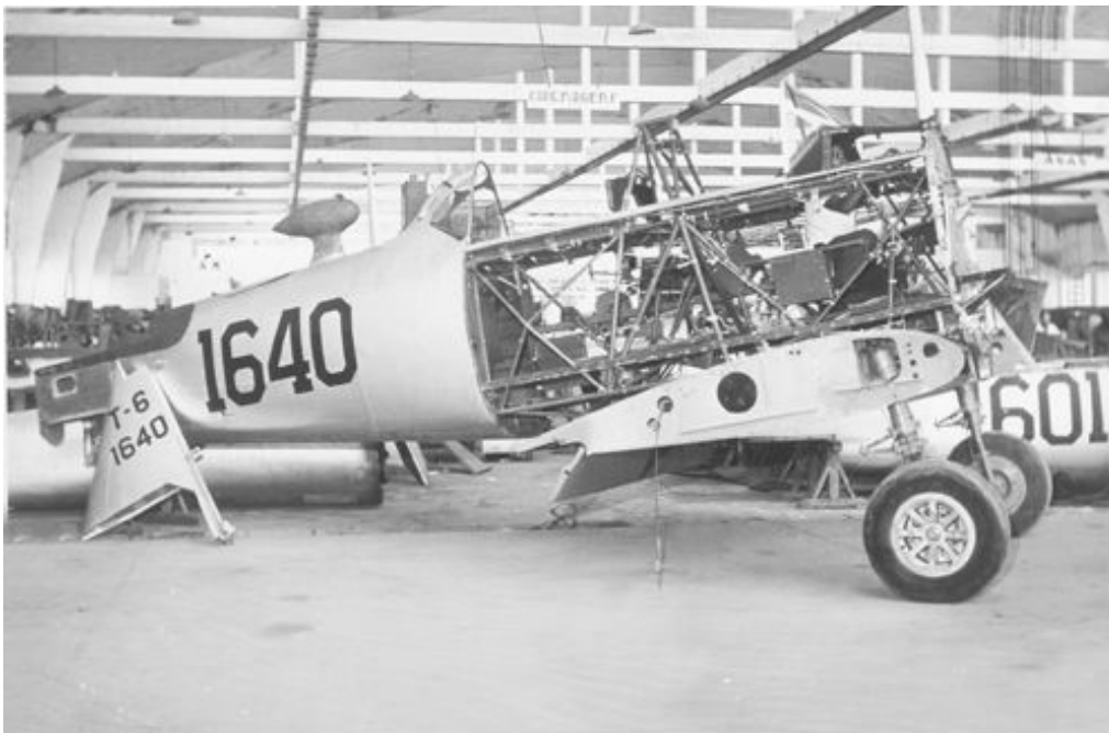
Fig. 22 – North American T-6 assembling line at Lagoa Santa plant.
