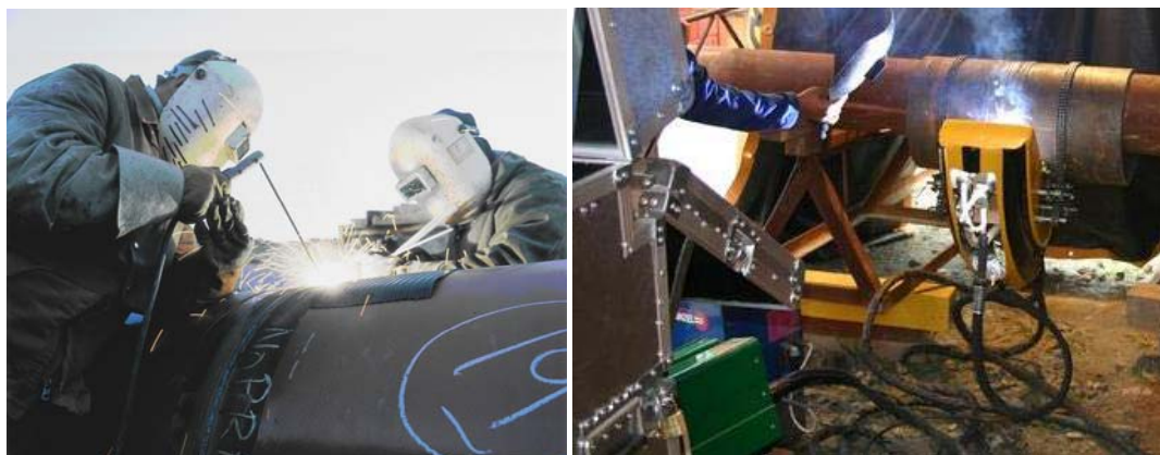
Figure 1: Manual welding of pipes and orbital weld robotic system.
