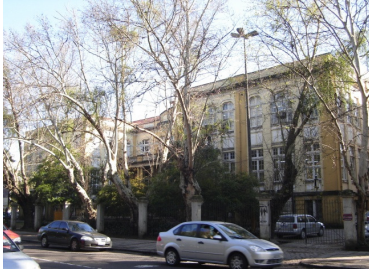
Figure 1. Building south façade
