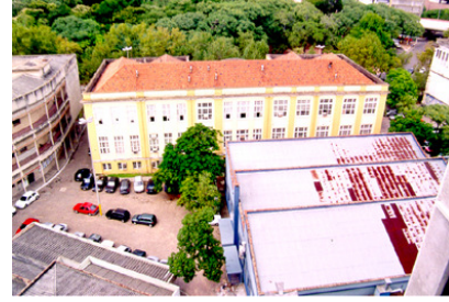
Figure 2. Building north façade
