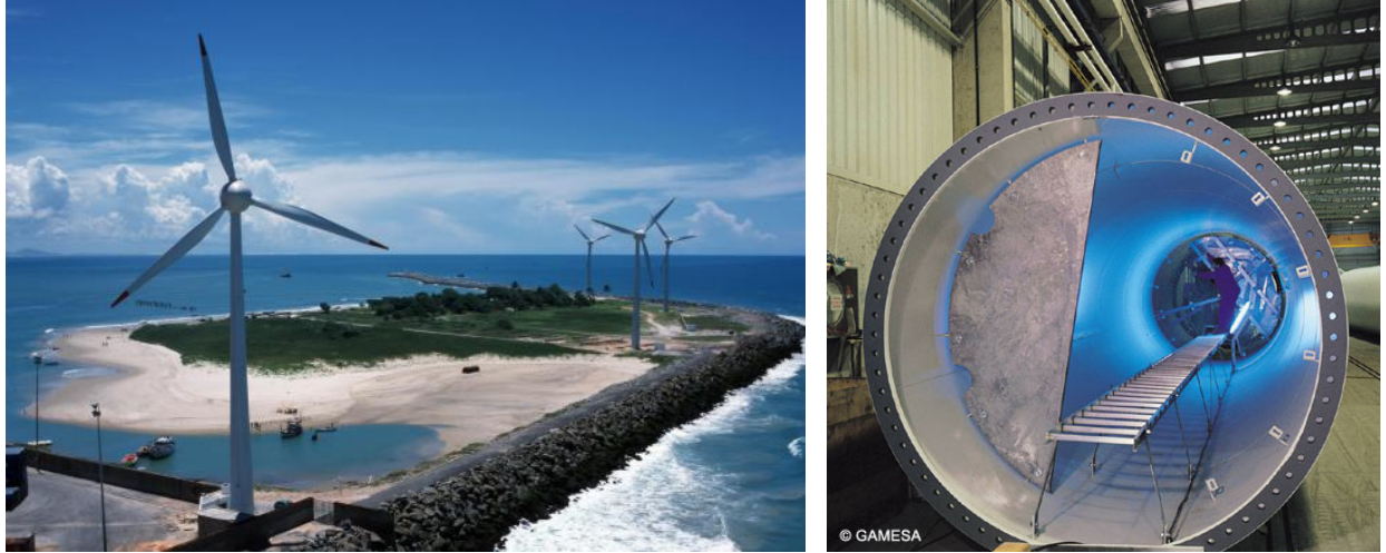
Figure 1. (a) Wind Park in Mucuripe/Ceará (Brazil, 2003): Four wind turbines E-40/600 kW (40 m rotor diameter). (b) Internal view of a conical steel tower in manufacturing.
