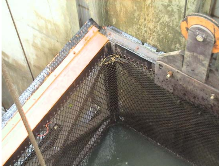
Figure 5. Rubber protection in the side of the chamber in order to avoid fish escape during its ascent
