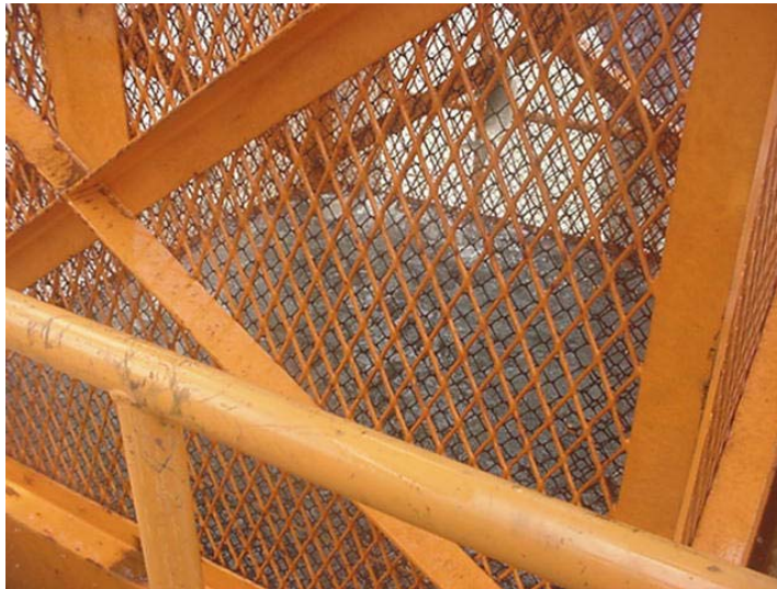
Figure 6. Flexible protection, inside the iron screen, to avoid fish injuries in the specimens jumping inside the chamber
