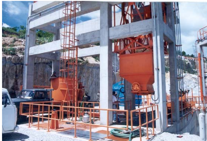
Figure 2. Santa Clara dam’s fish lift with a “trap and trucking” system
