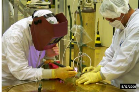
Figure 1. Titanium pipeline welding process
