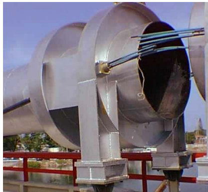
Figure 3. Stiffened ring support and anchorage of the cables
