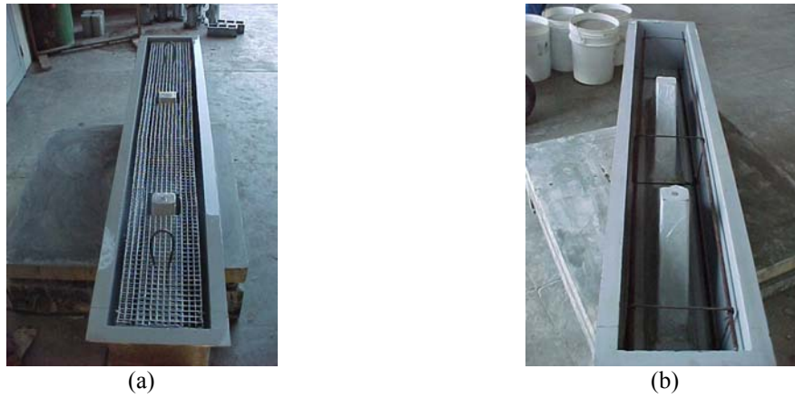
Figure 2. Fiberglass mold: (a) reinforcement cage and (b) reinforcement bars & stirrups.
