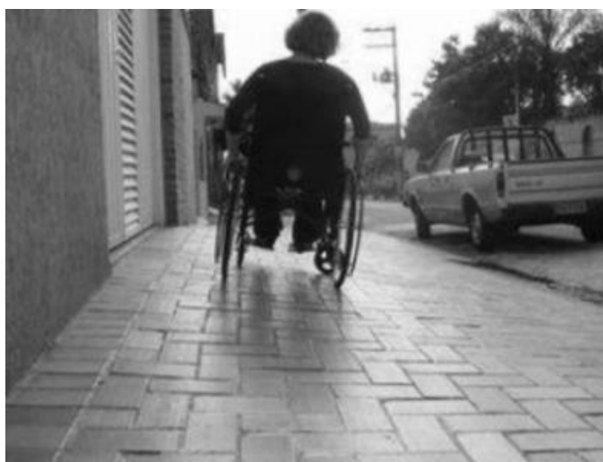
Figure 1 - A wheelchair user on a sidewalk with inadequate slope (Silva, 2009).
