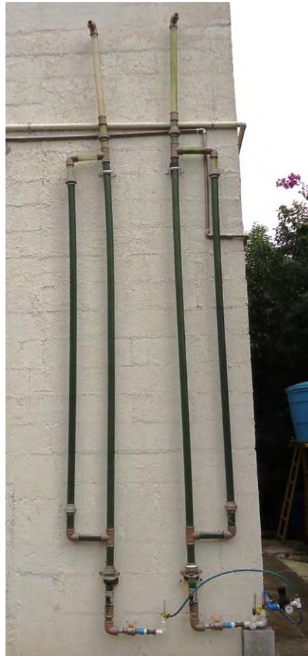
**FIGURE 03** - Air-Lift photobioreactors for cultivation of microalgae and CO<sub>2</sub> capture in biogas produced from the anaerobic digestion of waste.
