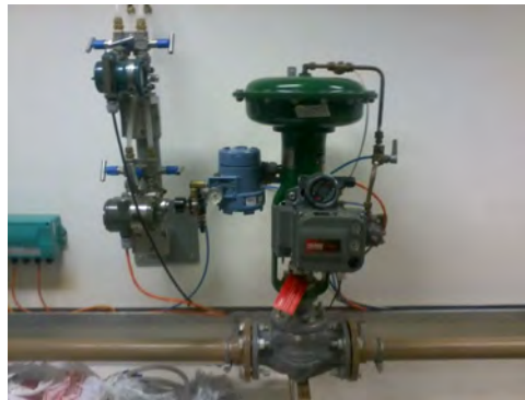
Figure 5. Teflon gasket valve
