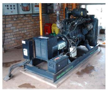
Figure 2. MWM 6.12T Gas Engine
