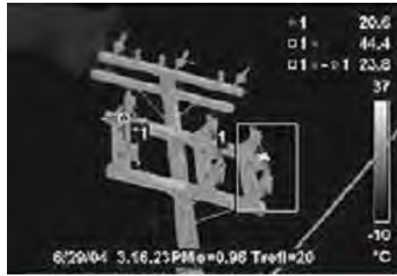
Figure 2. Inspection of elements aided by IR camera. Source: http://irisbuildingsciences.com
