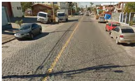
Figure 6. Type of track and street conditions of Jacob Lucchesi St.
