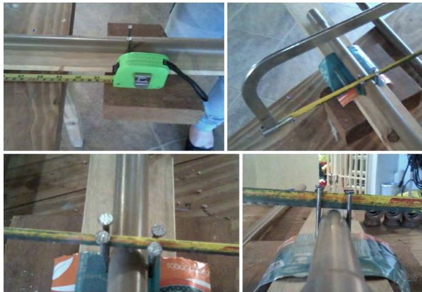
Figure 9. PVC pipes cutting (Author, 2012).
