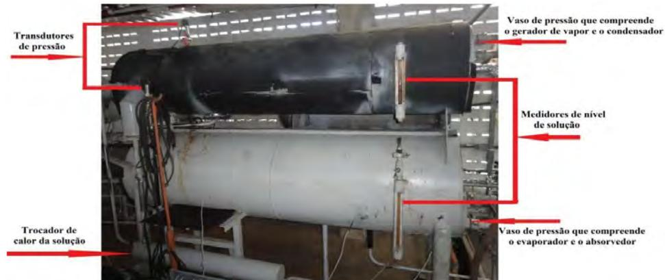
Figure 4 - Side view of the absorption refrigeration system IES-UFPB.
