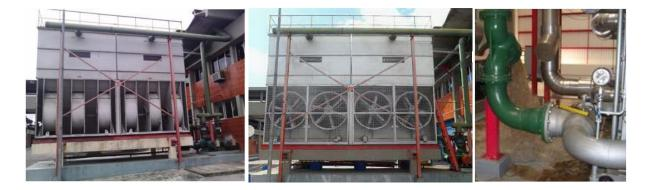
Figure 4. Reform of the cooling towers: (a) cooling tower before reform; (b) cooling tower after reform; (c) backwash in a plate and frame condenser
