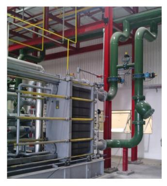
Figure 2. The plate and frame condenser used in the industry
