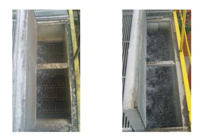
Figure 5. Distribution of water in spray nozzles before and after the reform
