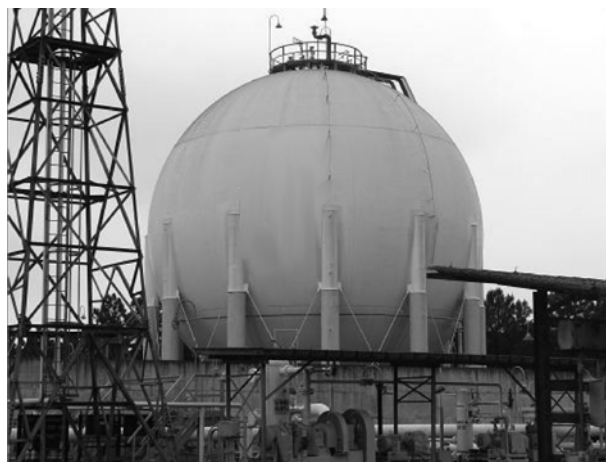
Figure 1. LPG storage sphere.
