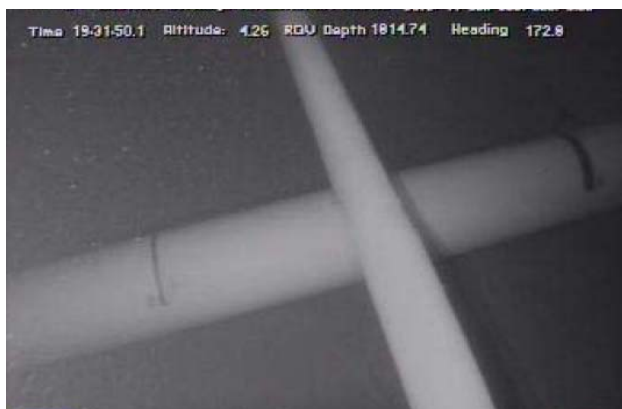
Figure 10 – PDET Pipeline Laid over a Sleeper in KP1.5.
