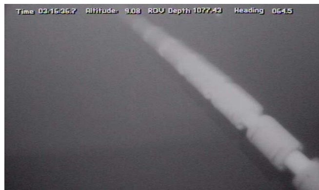
Figure 8 – Distributed Buoyancy Sections during Laying.
