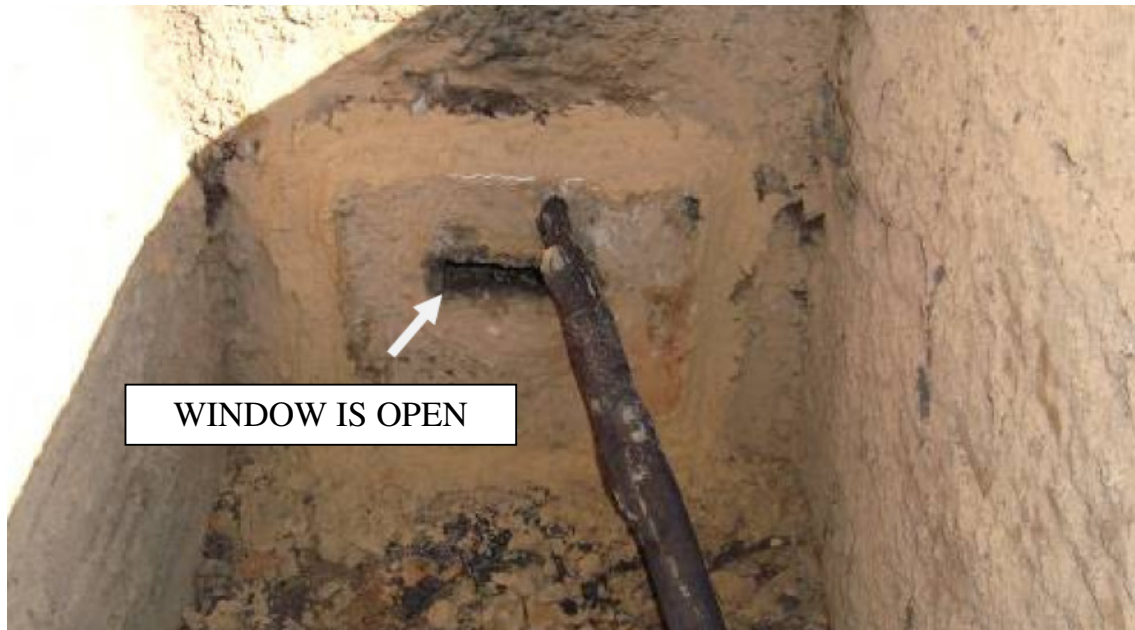
Figure 9. Air inlet during the cooling step
