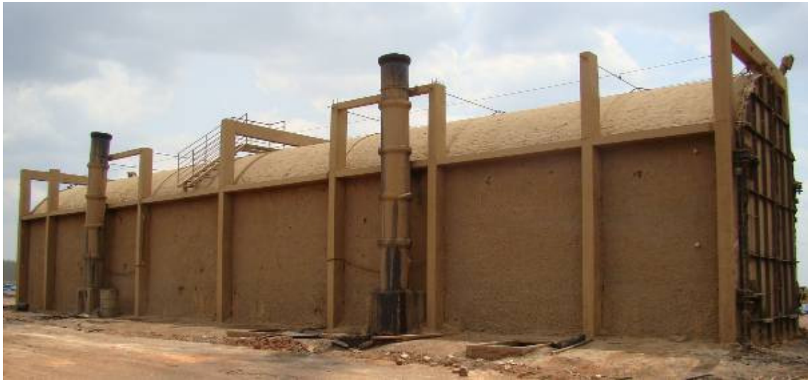
Figure 2. Typical rectangular kiln – RAC 220
