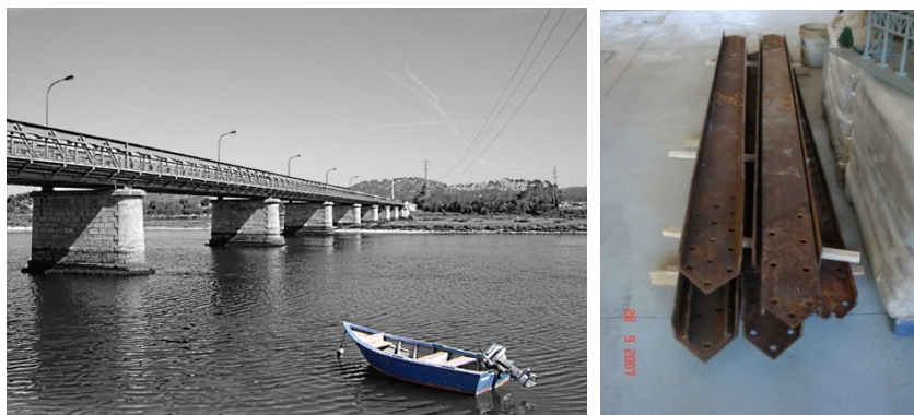
Figure 1. Fão bridge (left) and diagonals removed from the bridge (right).
