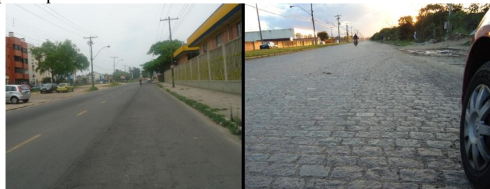
Figure 6. Asphalt pavement and cobble pavement.
