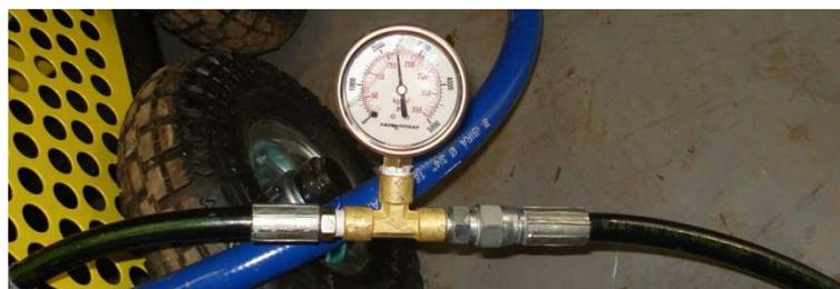
Figure 5. Manometer installed in the output of the hydrojet pump for pressure monitoring
