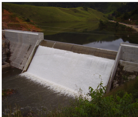
Figure 1. Uniform downstream flow over a stepped spillway
