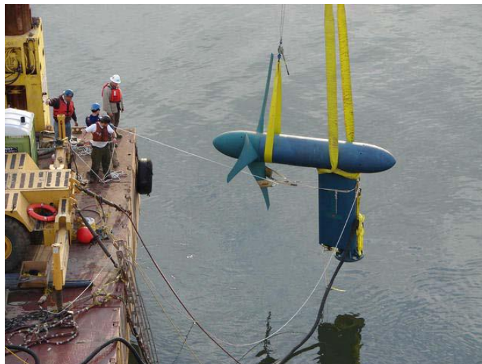
Figure 6. Hydrokinetic Turbine Verdant Power 35kW (Sale et al, 2009).
