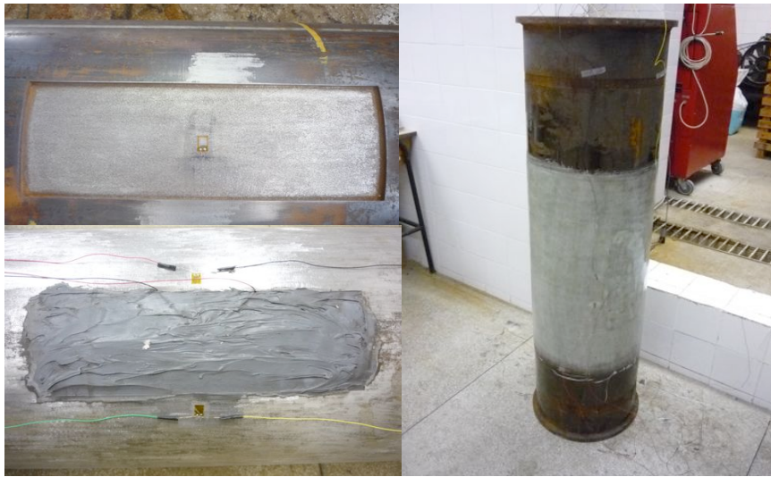
Figure 2. Composite sleeve installation
