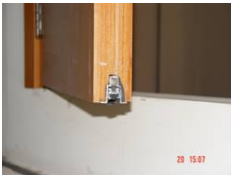
Figure 2. Views of Door 1, automatic door sealing system (a) and double door frame (b)
