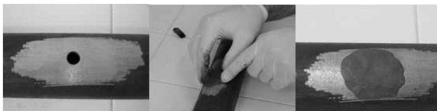
Figure 3. Epoxy repair procedure
