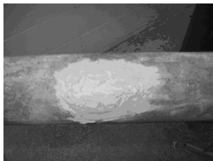
Figure 9. Epoxy Repair system C
