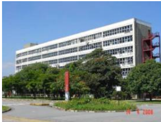
Figure 1. Front side of the University Administration building.
