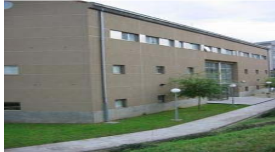
Fig.2. The new school (Paseo as Pontes).
