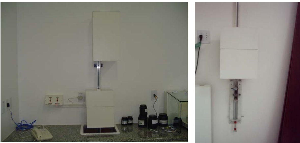
Figure 6. Elevator Box on the first floor, on the left. Elevator on the ground floor, with the inferior part without protection, on the right.
