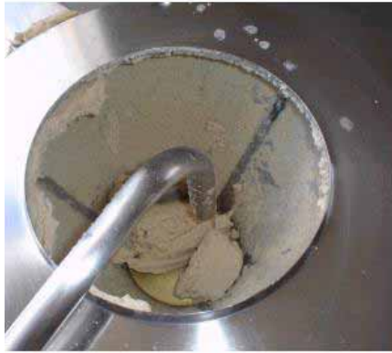
Figure 11. Filter condition after operation.
