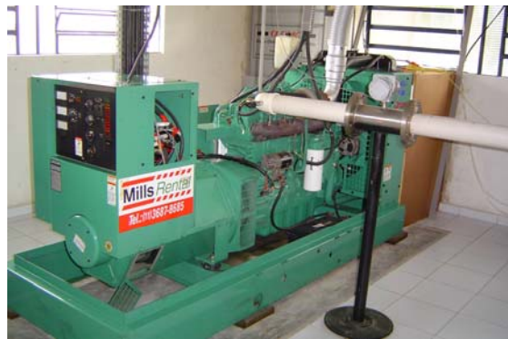
Figure 1. Diesel engine-Electrical generator system
