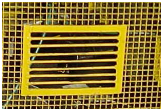
Figure 4. OP-20 – Raw material access grilles.
