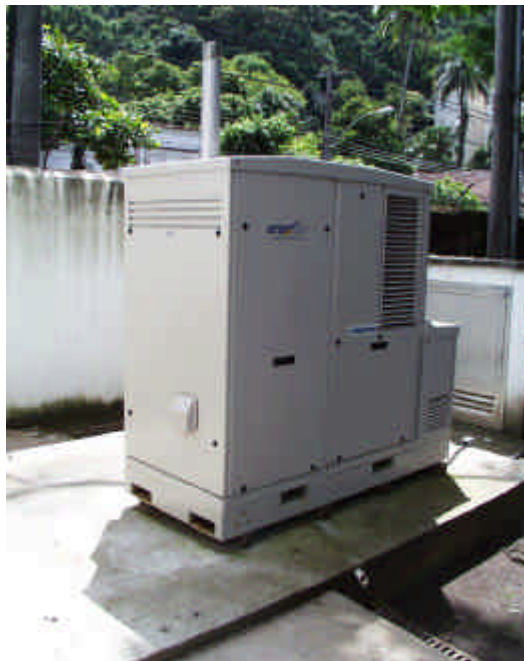
Figure 8. The 5 kW PEM type fuel cell at PUC-Rio
