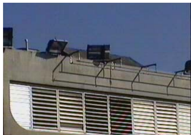
Figure 2. Details of the original structure.
