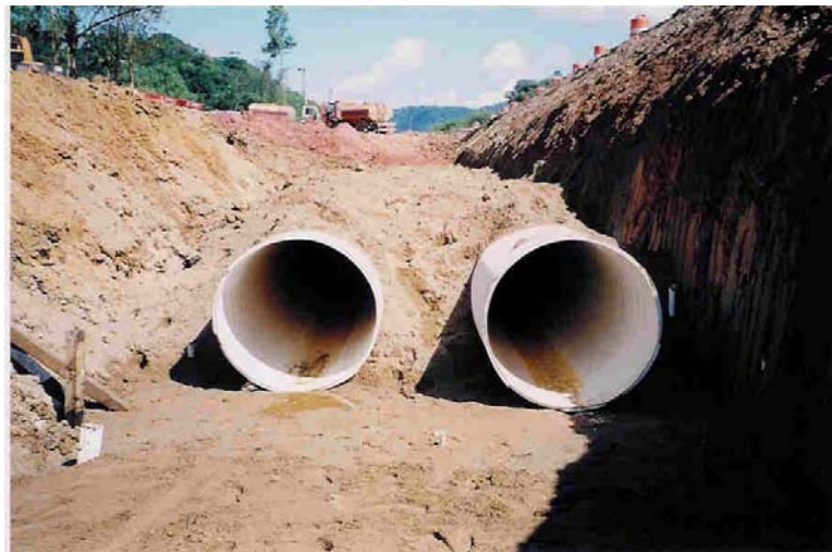
Figure 1. Underground pipes in drainage works
