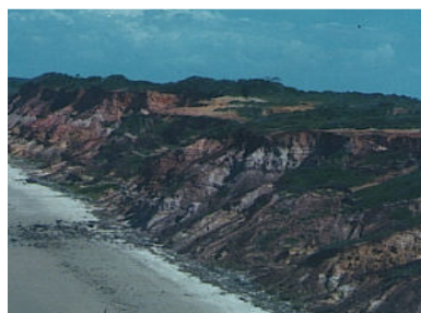
Figure 2. Coastal Cliff irregular structure.
