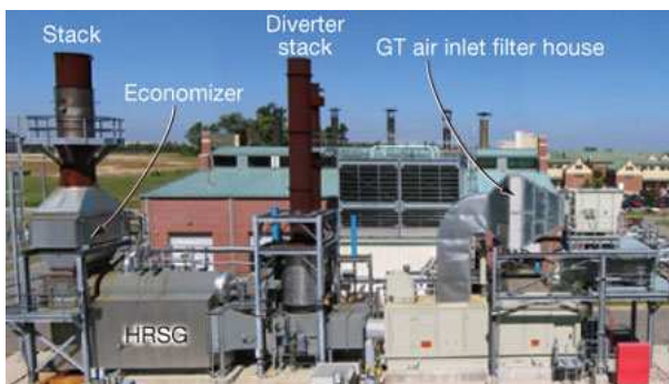
Figure 3: HRSG typical arrangement (Rentech Boilers) for a Solar Taurus 60 and the steam path diagram of an OTSG (IST)
