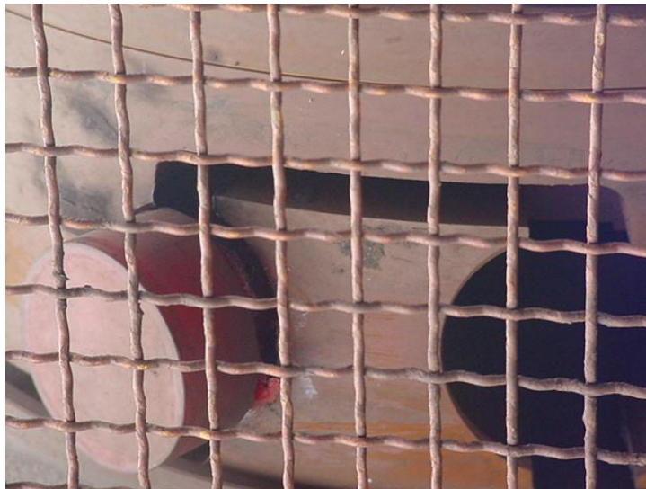
Figure 5. Release of an elastomeric element in service.
