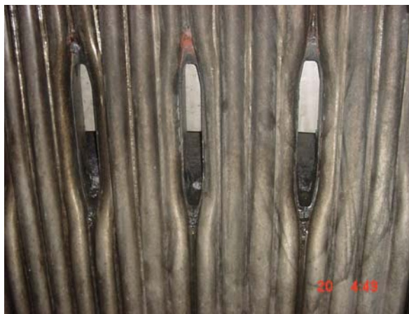
Figure 6. Primary air ports
